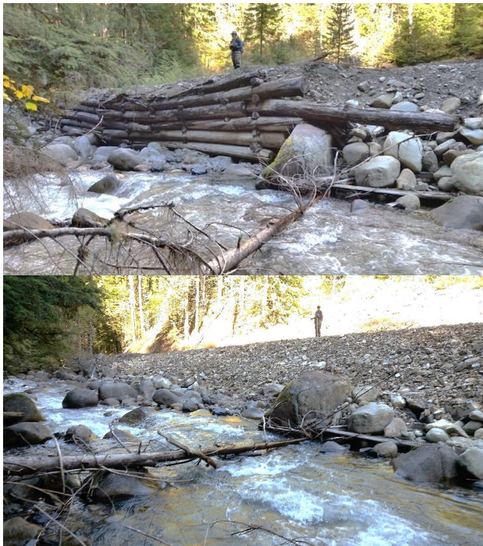
Figure 8. Unstable cribbing removal from Silverton Creek completed by Interfor (Top-Before-2015 and Bottom-After-2016).
